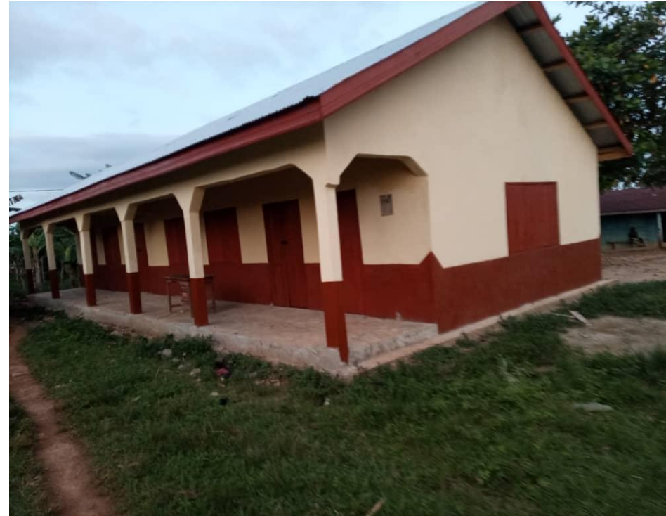
Completed 1No. 2-Unit KG block at Tumantu
