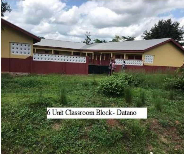
Completed 1No. 6-Unit classroom block at Datano
