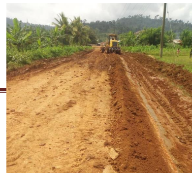
Reshaped 40km of road Districtwide
