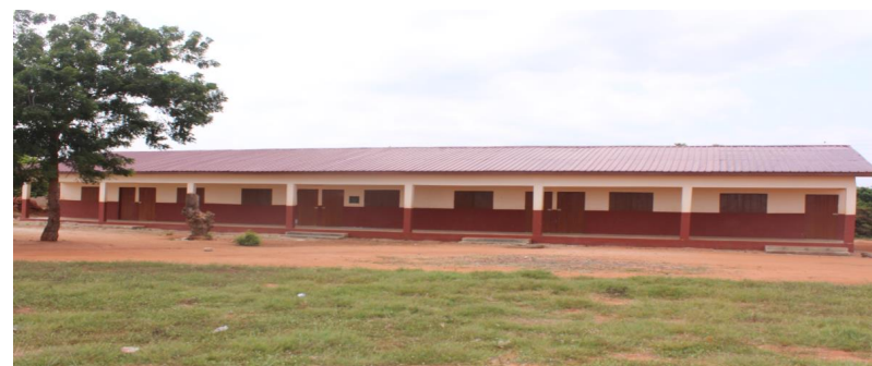
1No. 3-Unit Classroom Block at Agordeke
