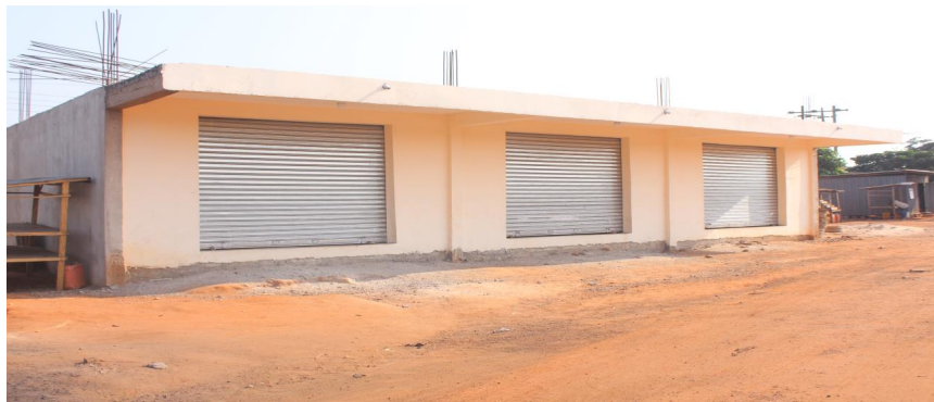
Lockable Stores at Dzodze
