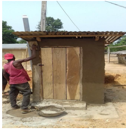
Figure 5: Completed Household Latrine
