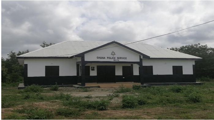
Figure 6: Police station at Wute
