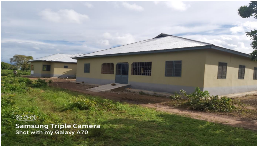
Completed Avosum CHPs Compound
