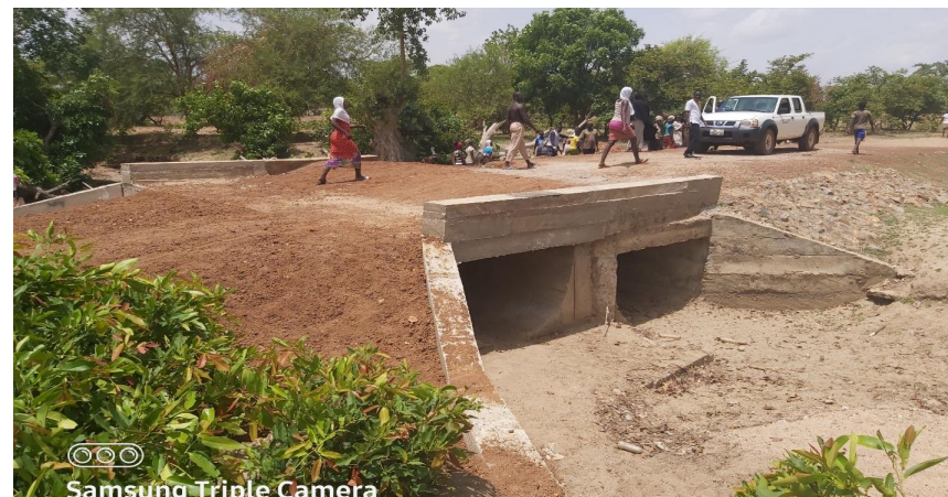
Construction of 1no. U Shape Culvert at Naate
