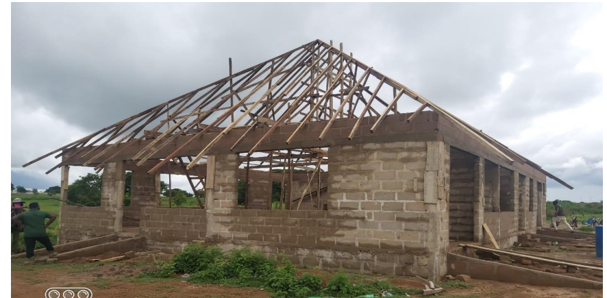
Construction of 1no. Slaughter House at Abilatega
