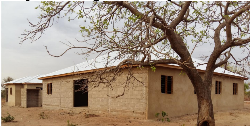
Completed Wadugu CHPs Compound
