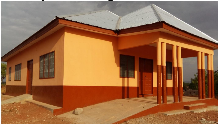
Maternity Block at Kugri Health Centre
