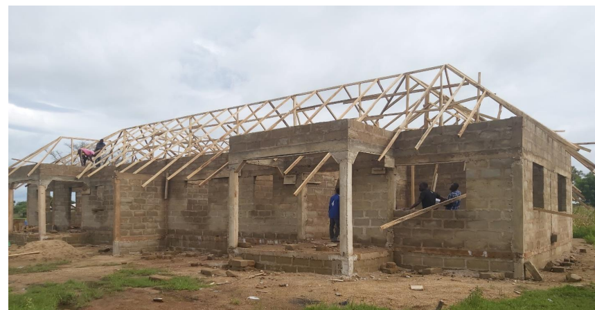
Construction of 1no. 2-Unit Seme-Detached Teachers Quarters at Sumanduri
