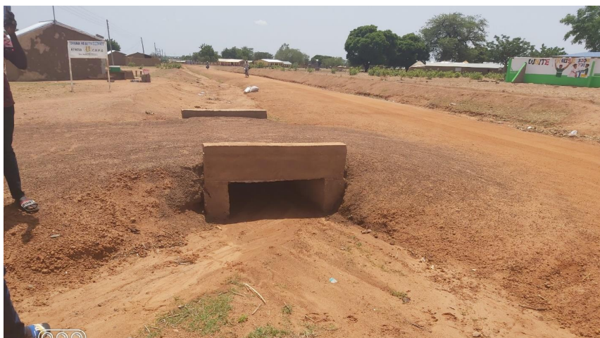
Construction of Culvert at Kpatia CHPs
