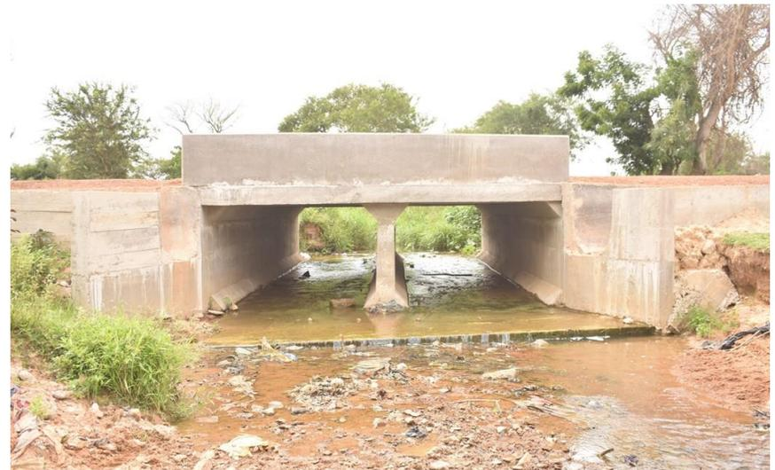
EMERGENCY CONSTRUCTION OF 2.5m x 1.5m DOUBLE BOX CULVERT WITH 0.9m U DRAINS AND APPROACH FILLING AT SOE NEW TOWN
