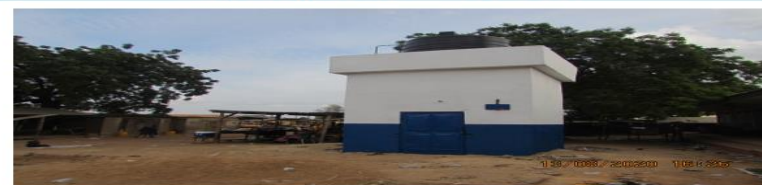
Drilling and mechanization of 3No. Boreholes at Zebilla, Binaaba and sapeliga market as means to curb covid-19.
