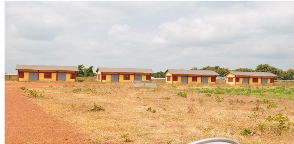
• 4No. Yam Storage Constructed at Kpassa New Market
