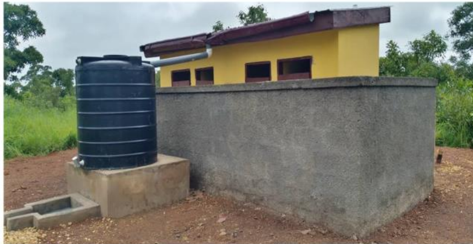
1NO. 4SEATER KVIP CONSTRUCTED AT KOFINYI
