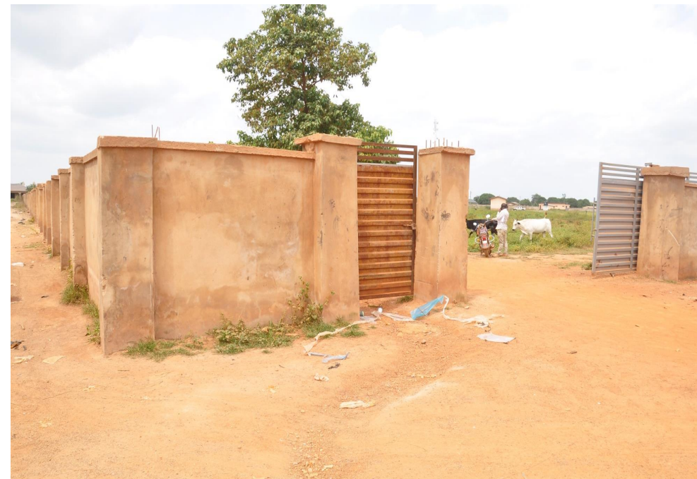
• Fenced 1.6km-Lengh X 2.1m Height Wall Of Kpassa New Market
