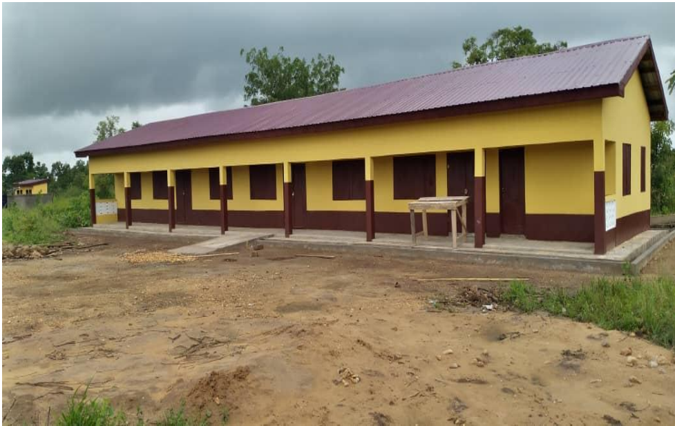
• 1 No. 3 Unit Classrooms Block Constructed
