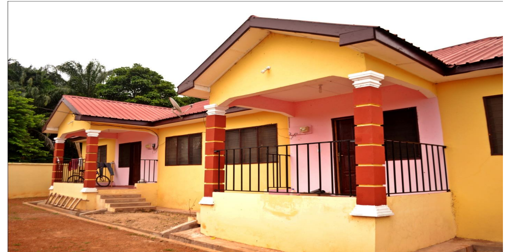
8. Construction of 2-semi-detached nurse's quarters at Comfort Offodie Health Center at Nkonya - Kadjebi
