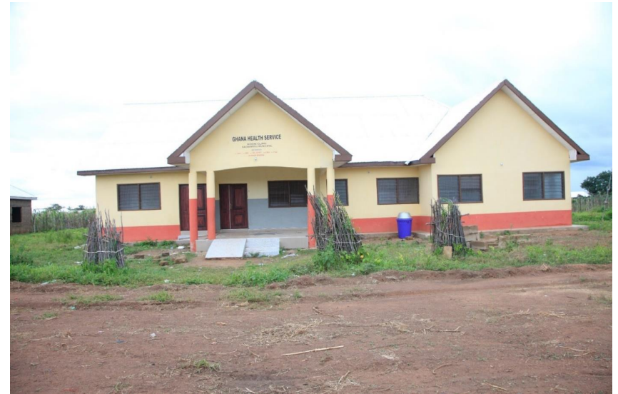
Figure 1 Construction of Clinic at Kogni- DDF
