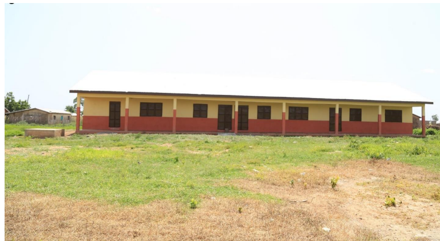
Figure 4 Constructed and Furnished 1no. 3unit Classroom and Ancillary Facilities at Kasalgu
