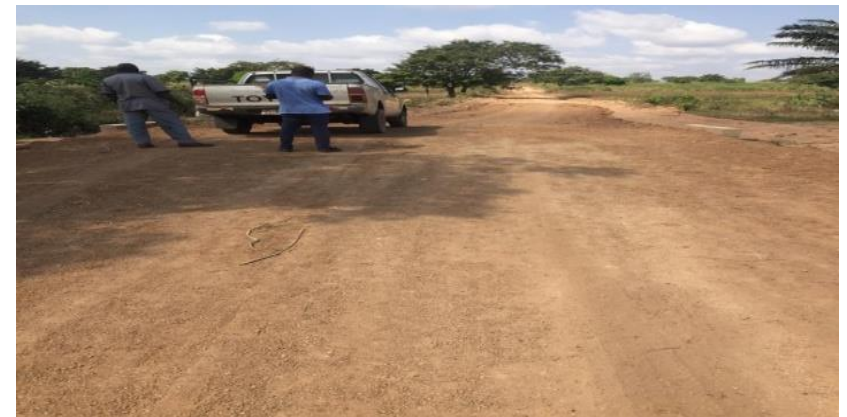
Figure 7: Rehabilitation of Nyankpani-Wumbejado (3.5 km) , Jilo-Kukuo & Nyankpani-Yadoya Feeder Roads
