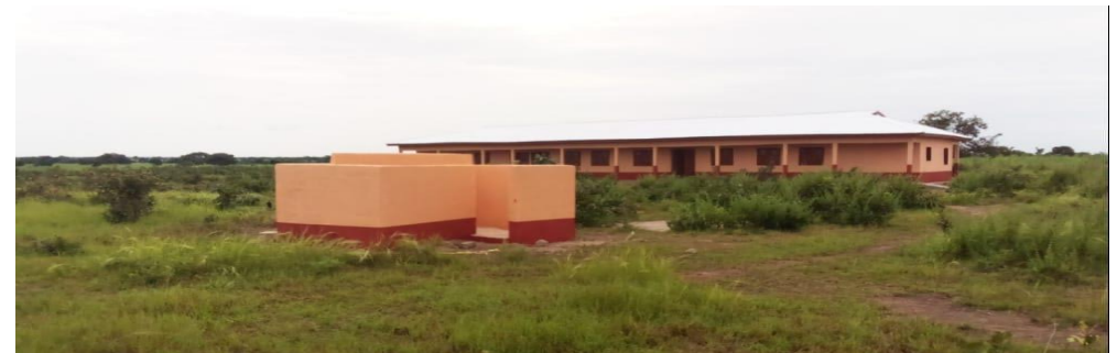
Completed and furnished 3unit classroom block at Duuni
