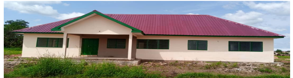
Completed Teachers Quarters at Gambaga
