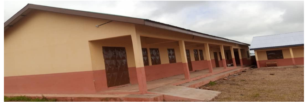
Completed and furnished 3unit classroom block at Gambaga
