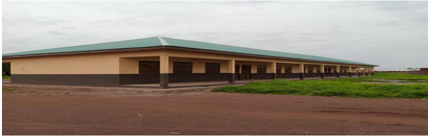
Completed and furnished 3unit classroom block at Gbintiri
