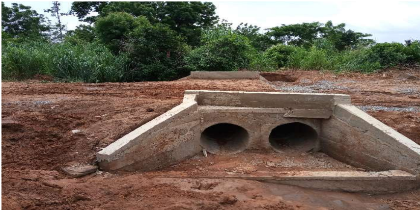
Constructed 2No. Culvert at Ahinase and Mota
