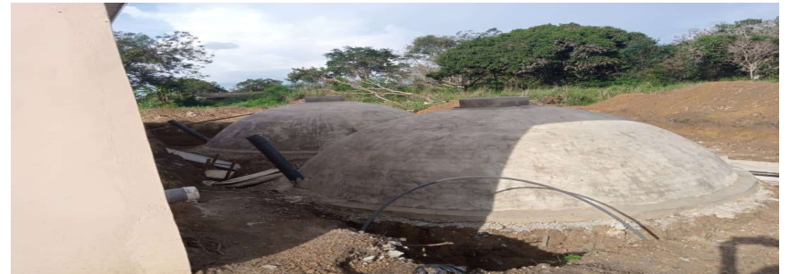
Completed 1No. 6-Seater W/C toilet with Bio-digester at Abetifi Ridge School
