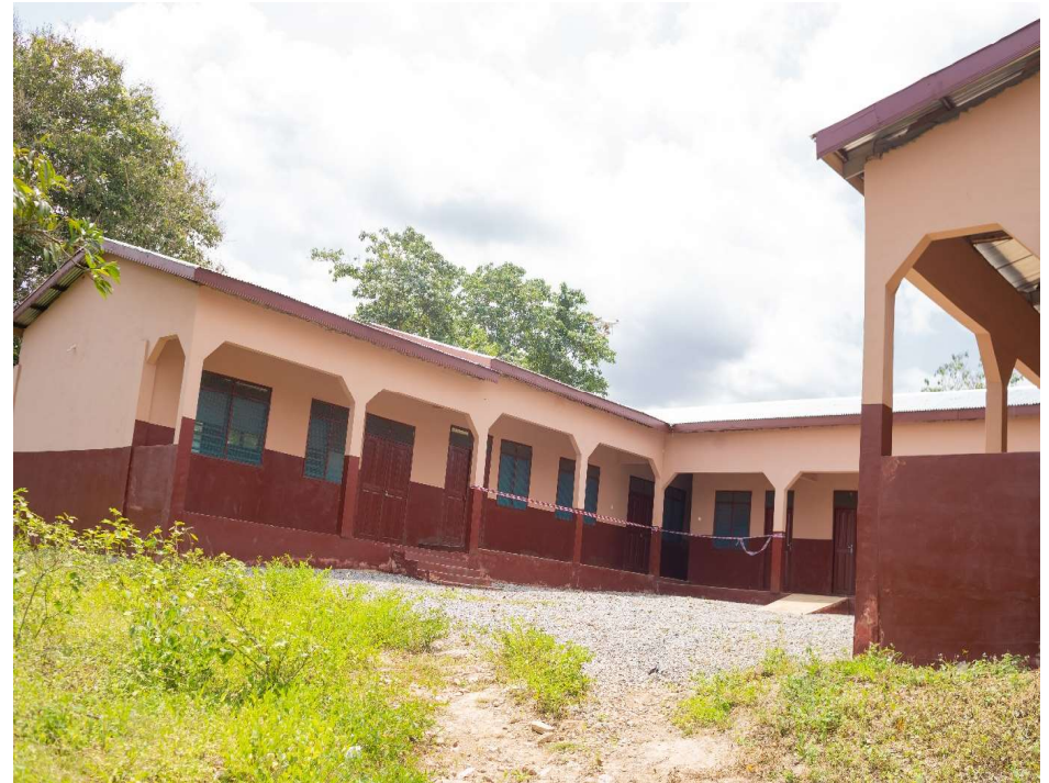
1 No. 6-Units Classroom Block @ Dokyi
