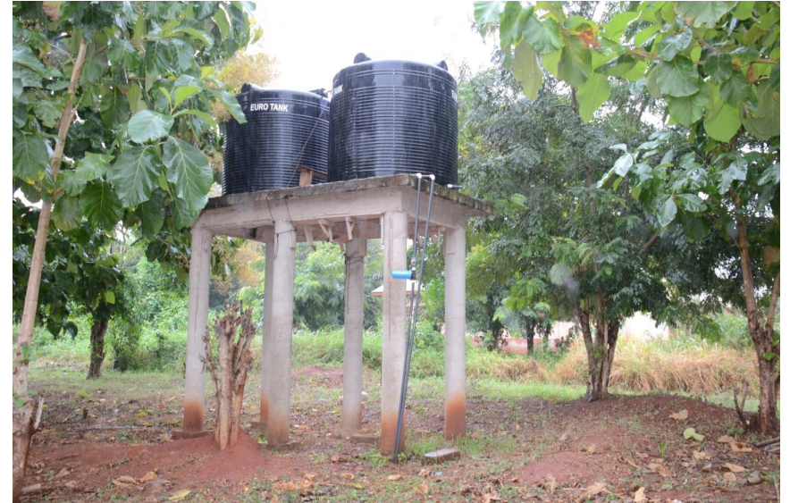
High reinforced concrete stand
