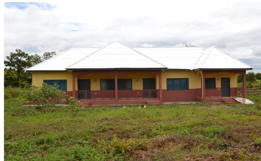
Branam CHPS Compound
