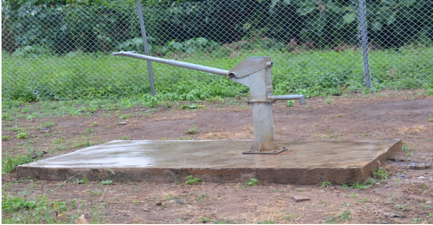
Borehole fitted with Hand pump at Botenso
