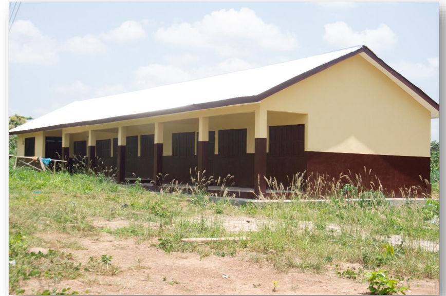
6. 3-UNIT CLASSROOM BLOCK WITH ANCILLARY FACILITIES CONSTRUCTED AT ABRONYE (FUNDED BY DDF)
