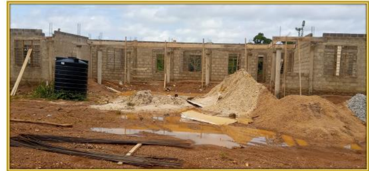
• CONSTRUCTION OF 1NO. 6-UNIT CLASSROOM BLOCK @ DABAABI • {DPAT}
