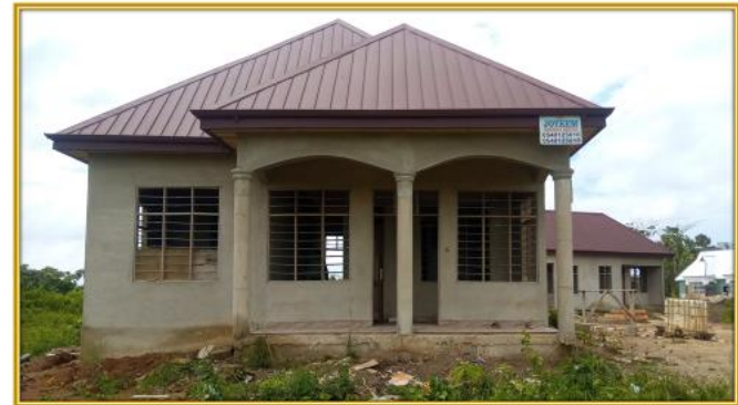
• CONSTRUCTION OF 1NO. CHPS COMPOUND @ ATESIKROM • {DACF}
