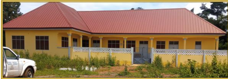
• CONSTRUCTION OF 1NO. KG BLOCK WITH ANCILLARY FACILITIES @ GYEDIEM • {DPAT}
