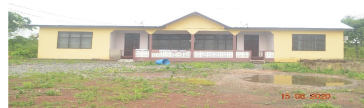
REHABILITATED 1NO. 6 UNIT CLASSROOM BLOCK AT DAMA NKWANTA (DACF)
