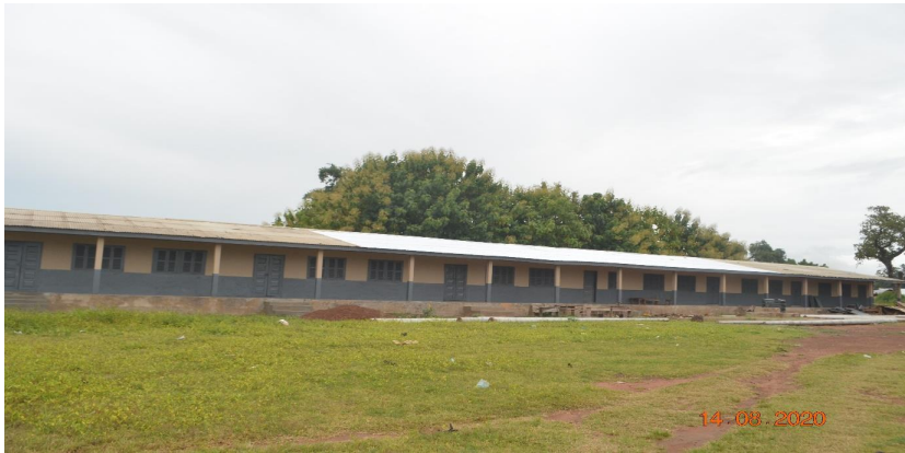
CONSTRUCTED OF 1NO. HEALTH CENTER AT DAMA NKWANTA (DDF)
