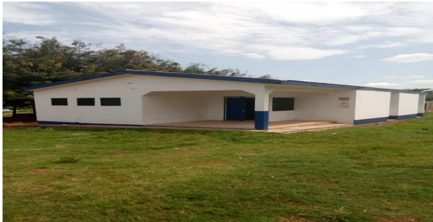
BUSINESS ADVISORY CENTRE (B.A.C) OFFICE AT JEMA RENOVATED
