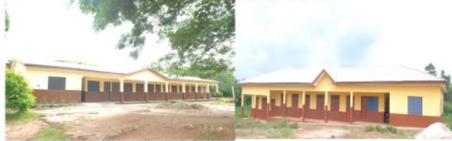
CONSTRUCTED 100 UNIT CLASSROOM BLOCK WITH OFFICE, STORE, STAFF COMMON ROOM AND ICT ROOM AT AKOKBASSO
