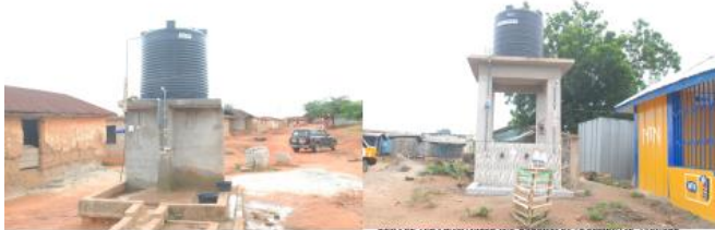
DRILLED AND MECHANIZED 100 BOREHOLES AT SENCHI, ATTAKROM AND SUTAM
