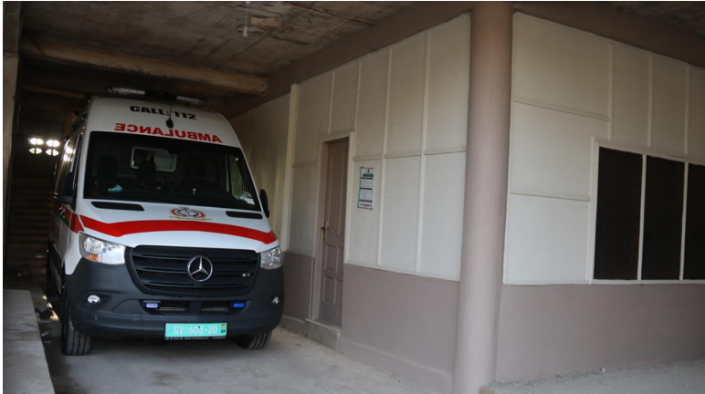
3-Offices for National Ambulance Unit has been completed at Tafo Community Centre
