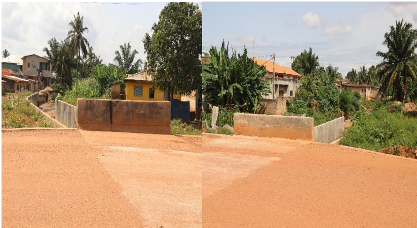
Culvert Bridge has been constructed at True Vine Junction, Boanwene
