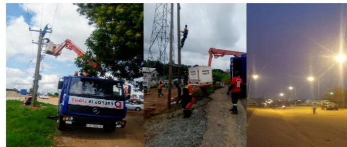
Supplied and Installed Underground Cables and Street Lights within the Municipality
