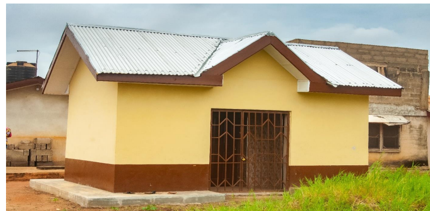
Completed Urinal at Deduako
