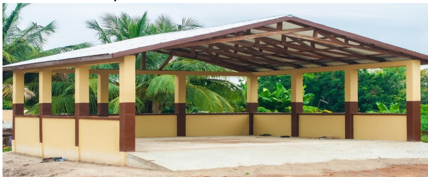
Constructed 1No. Skip Pad at Bebre
