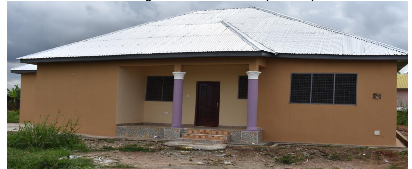
1No. 3 Bedroom Doctors Bungalow at Asonomaso Hospital Completed
