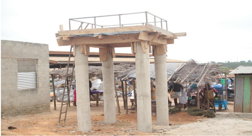
MECHANISED BOREHOLE WITH EXTENDED STAND PIPES-BOMFA
