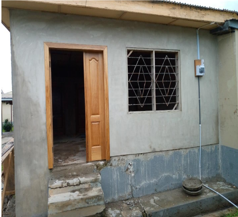
CONSTRUCTION OF AN ISOLATION CENTER AT JUABEN HOSPITAL
