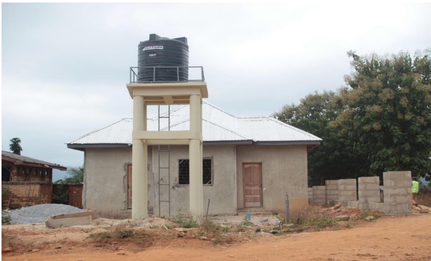
16-SEATER WC AND 4-URINAL FACILITY WITH A MECHANISED BOREHOLE AT ACHIASE
