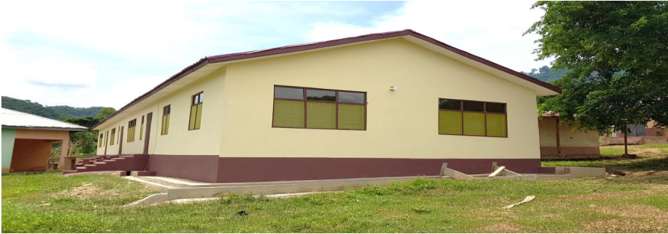
CONSTRUCTED OF 1 NO. 3 UNIT JHS CLASSROOM BLOCK WITH OFFICE, STORE AND LIBRARY
