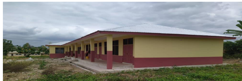
CONSTRUCTION OF 1NO. 12-SFATER WC TOILET AND MECHANISED BOREHOLE AT KOKOFU b). CONSTRUCTION OF 1NO. 6 UNIT CLASSROOM BLOCK WITH ANCILLARY FACILITIES AT ANWIAM AMENASE IN USE.
