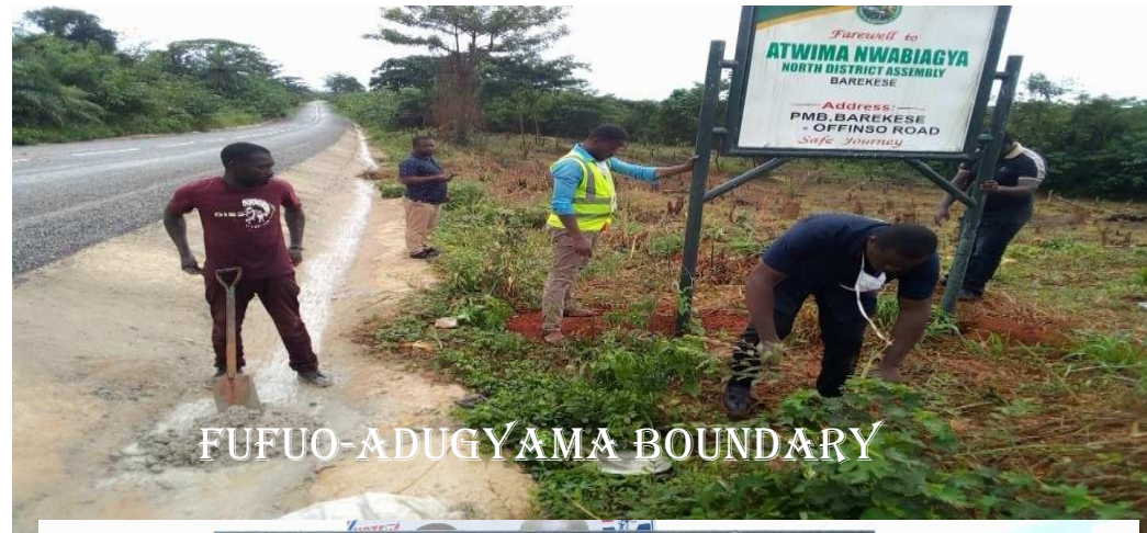
FABRICATION AND INSTALLATION OF 8 Nos. BOUNDARY SIGN POSTS FOR ANNDA
