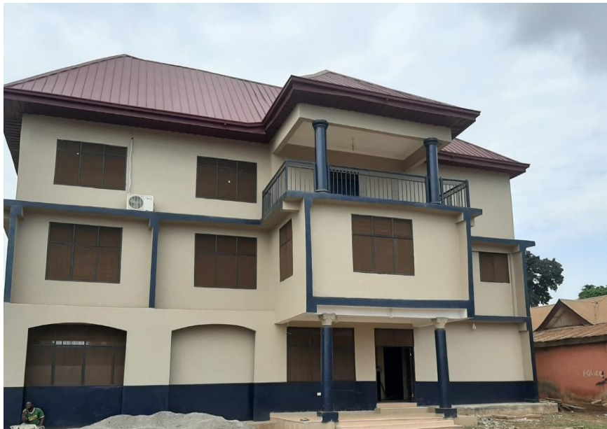
Constructed of 2-Storey Police Station at Abuakwa
