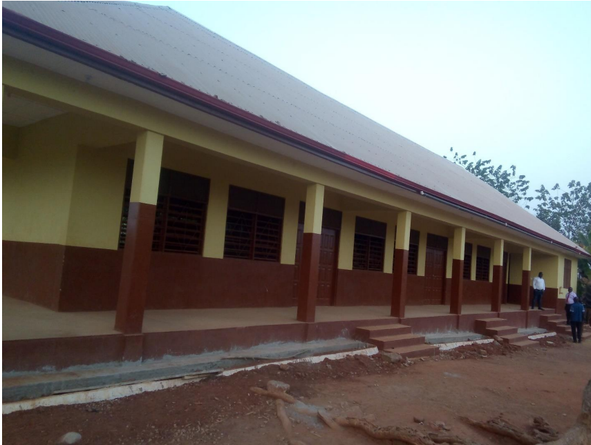
Constructed 1no. 3-unit classroom block at Kyereyaase
