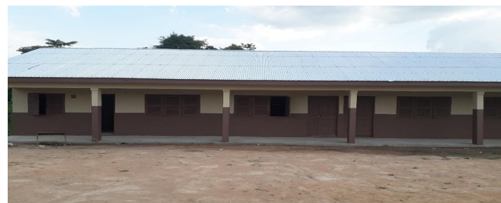
6-Unit classroom block with auxiliary office at Menam
