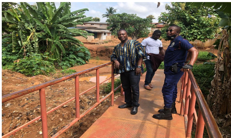
CONSTRUCTED STEEL BRIDGE AT AGOGO ZONGO
