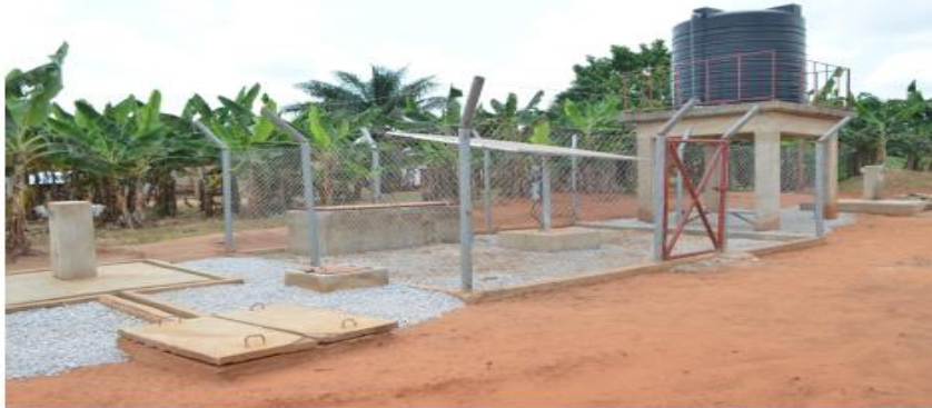
COMPLETED 1 NO. SOLAR POWERED MECHANIZED BOREHOLE LOCATION: ABOSOMTWEAGYA
