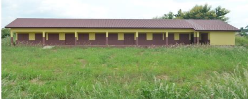
COMPLETED 3- UNIT CLASSROOM BLOCK WITH ANCILLARY FACILITIES LOCATION: ATUNSU
