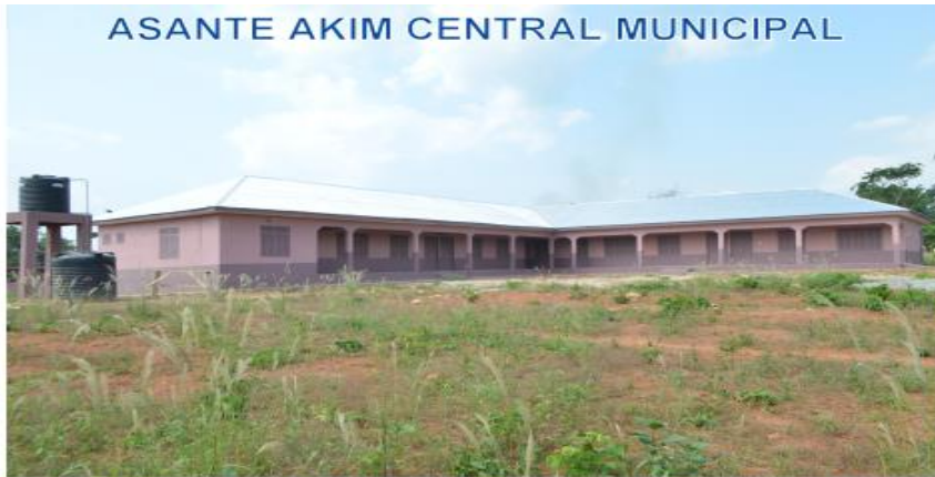
COMPLETED 1 NO. 5 UNIT KG AND LOWER PRIMARY CLASSROOM BLOCK WITH ANCILLARY FACILITIES, 5 SEATER SQUAT WC TOILET WITH MECHANIZED BOREHOLE AND OVERHEAD TANK AND SUPPLY OF FURNITURE AT KYEKYEWERE
