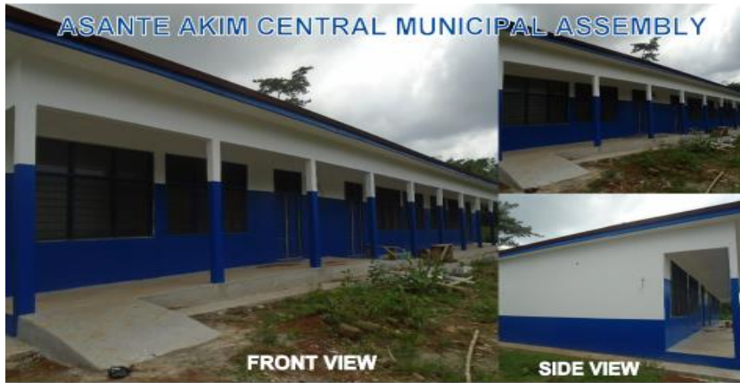
3 UNIT CLASSROOM BLOCK AT WESLEY HIGH SHS
