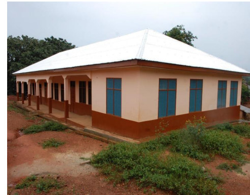
Constructed and Furnishing of 3-unit Classroom Block with Office, Store, Staff Common Room, 4-Seater KVIP and 2-Unit Urinal at Ahwerewam R/C Primary School (Funded by: DPAT)
