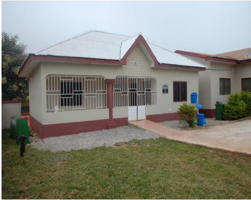
Constructed of 1 NO. 2 Bedrooms (Covid-19) Isolation Center with Nurses post Toilets with bath at St Edwards Hospital, Adugyama (DPAT)
