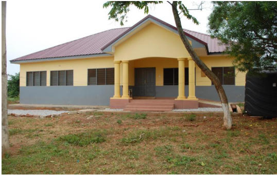
Constructed of Maternity Block, Changing Room, Store, ANC, Delivery Room and Lay-In-Ward at Pokukrom Health Centre (DDF)
