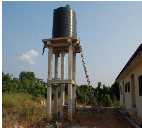
Constructed and Mechanization of 1 NO. Borehole at Adugyama Teacher's at Adugyama Teachers Quarters (Founded DDF)
