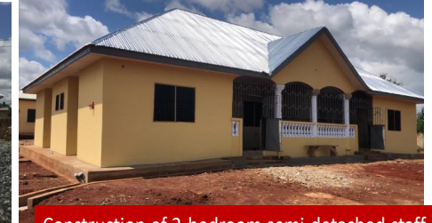
Construction of 2-bedroom semi-detached staff quarters at Duayaw Nkwanta
