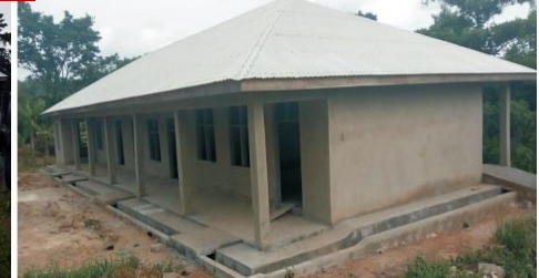
Construction of 1no. 3-unit classroom at Tanokrom
