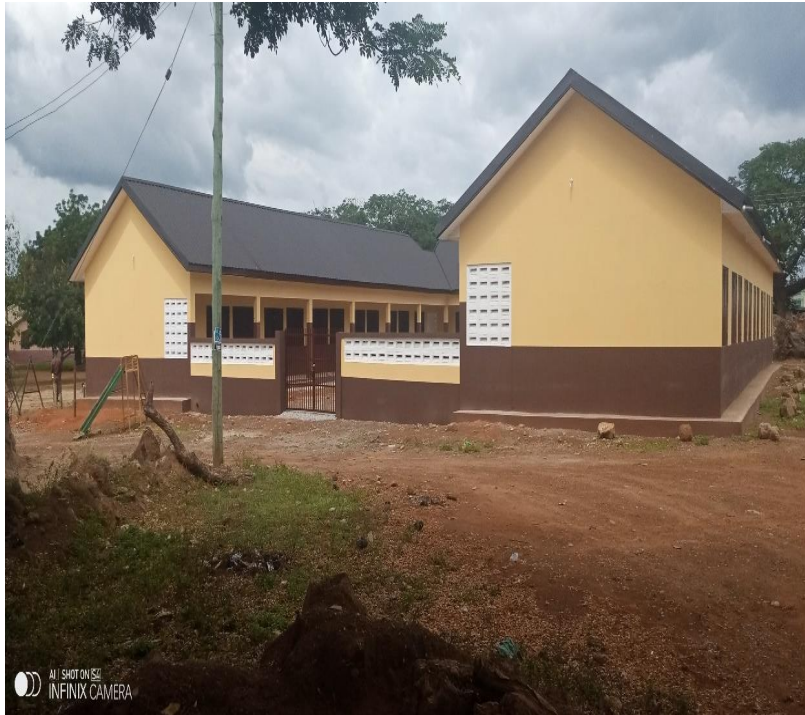
CONSTRUCTION OF 10NO. 6-UNIT CLASSROOM BLOCK WITH ANCILLARY FACILITIES IN THE MUNICIPALITY
