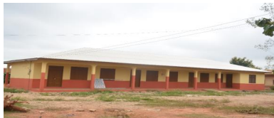
Construction of 3no. 3-unit classroom block with ancillary facilities at Duayaw Nkwanta R/C, Subonpang and Adrobaa
