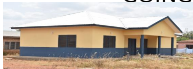
Construction of Police Post at Tanoso
