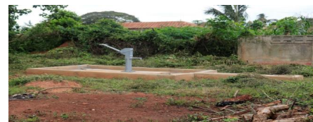
Drilling of 10no. Boreholes Fitted with Hand pump
