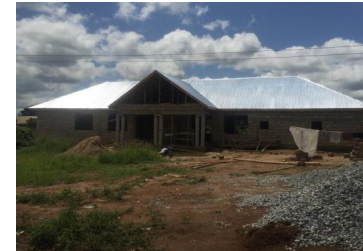
Construction of Hostel facility at Yamfo College of Health
