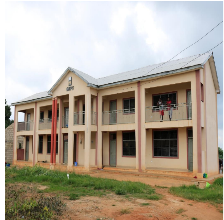
CONSTRUCTION OF 1 STOREY MALE HOSTEL FACILITY AT ST. JOHN OF GOD COLLEGE OF HEALTH AT DUAYAW NKWANTA
