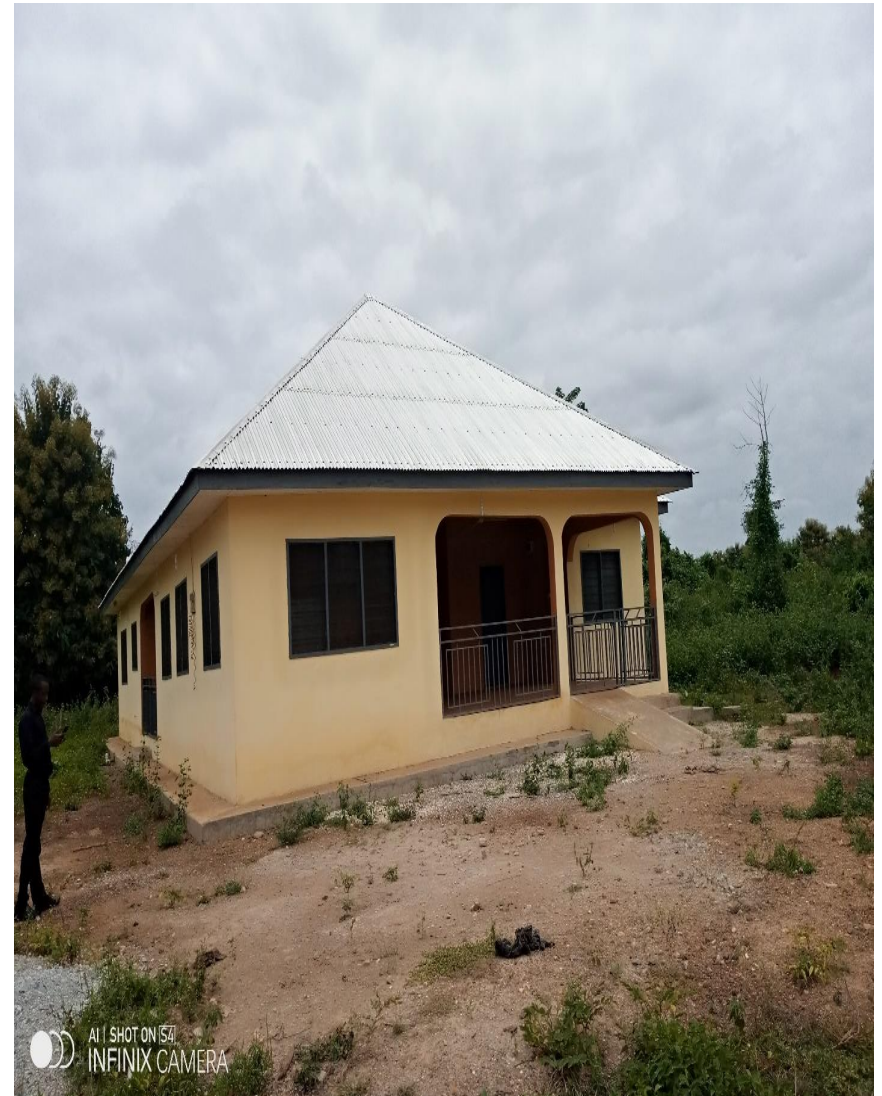
1 No. CHPS Constructed at Atudrobese
