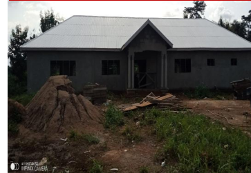
Construction of Hostel facility at Tanoso CHNTS
