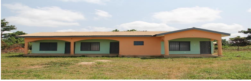
Construction of CHPS Compound with Ancillary Facilities at Yaw Owusukrom
