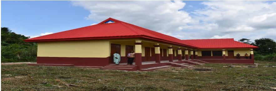
Construction of 16 seater Aqua Privy Toilet at Goamu Koforidua
