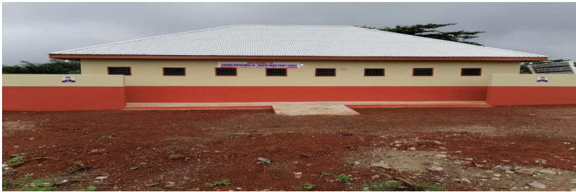
Construction of 1No. 4Unit Nurses Quarters at Biaso
