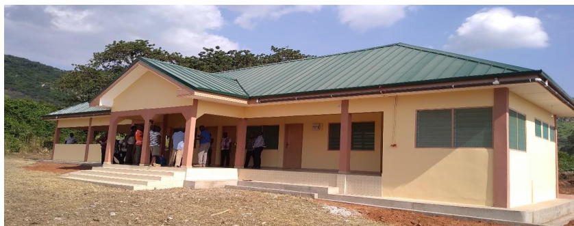
Completed CHPS Compound in Kpongbonikope
