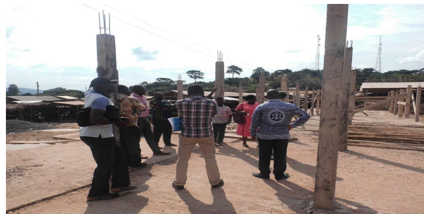
2No. Market Shed at Kpeve Market
