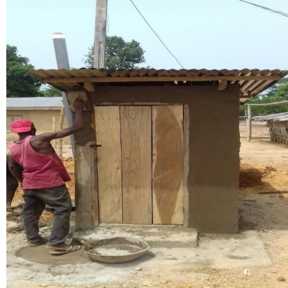
Figure 5: Completed Household Latrine
