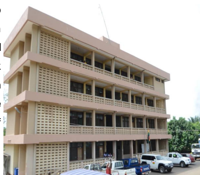
Figure 2: Hohoe Municipal Main Administration
