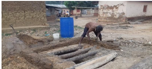
Figure 6: Household Latrine under Construction
