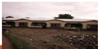
RENOVATION WORK ONGOING, STAFF QUARTERS B, FUNSI
