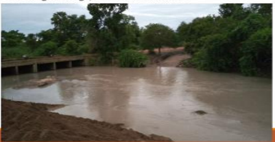
Desilting of Bridge, Funsi-Wahabu Road
