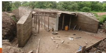
Construction of Culvert, Gbantala
