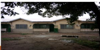
RENOVATION WORK ONGOING, STAFF QUARTERS A, FUNSI
