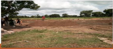
3 UNITS CLASSROOM BLK, GUONO (WIP)
