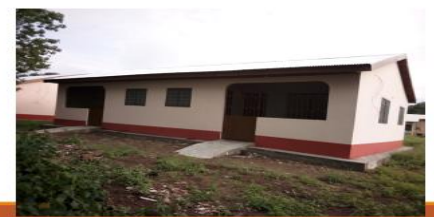
CONSTRUCTION OF SEMI-DETACHED STAFF BANGALOW, FUNSI
