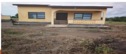
CONSTRUCTION OF LABOUR WARD AT BUFFIAMA
