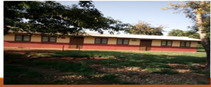
RENOVATION OF 6 UNITS CLASSROOM BLOCK, MANWE
