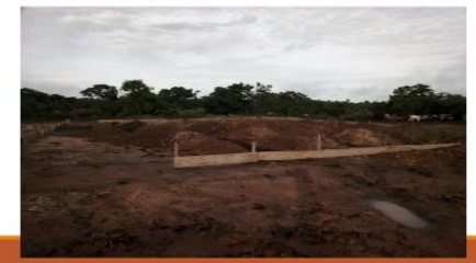
CONSTRUCTION OF DISTRICT HOSPITAL WARDS, FUNSI
