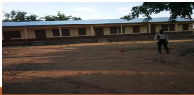
RENOVATION OF A 3 UNIT CLASSROOM BLK, KPALINYE.
