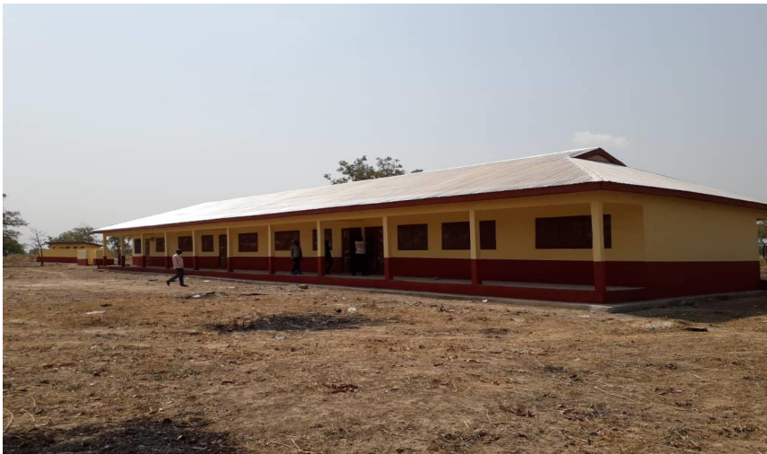
Figure 4: 1 No. 3-Unit Classroom Block at Chamba JHS
