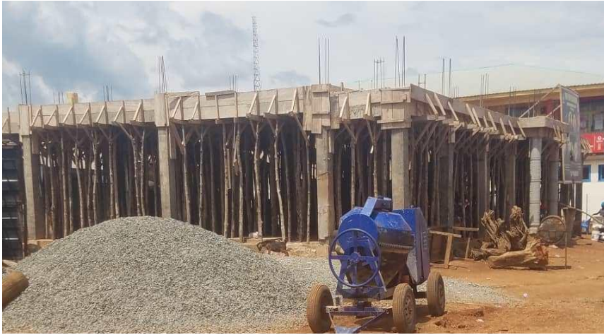
Figure 3: 1 No. 24-Unit Market Storey under Construction
