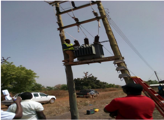
Figure 4: Gumonaayili Electrification project
