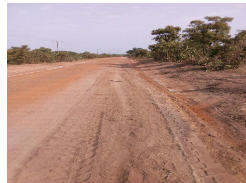
Figure 7: Reshaping of Digbila-Galwei Road
