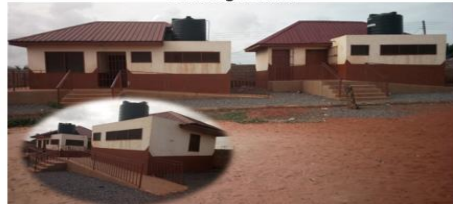
Project Description: Improved Institutional Sanitation & water supply at Tema East – Manhean S.D.A Basic School Digital Address: GK-0066-3656 Funding : GAMA
