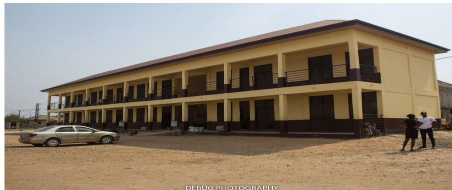
CONSTRUCTION OF 2 STOREY 6 UNIT CLASSROOM BLOCK AT KUBEKRO
