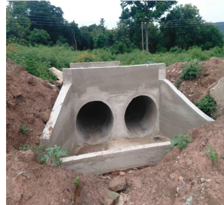
Constructed 1No. Culvert at Nkwantanang and Ahinase Junction to Nkwantanang Feeder Road reshaped
