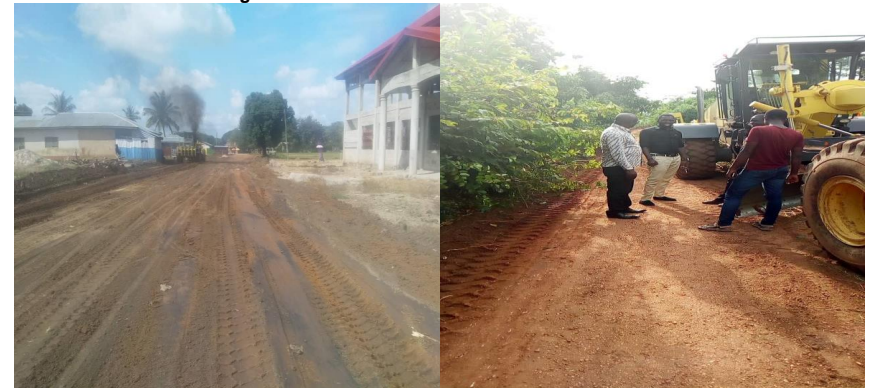
Figure 6 RESHAPING OF FEEDER ROADS
