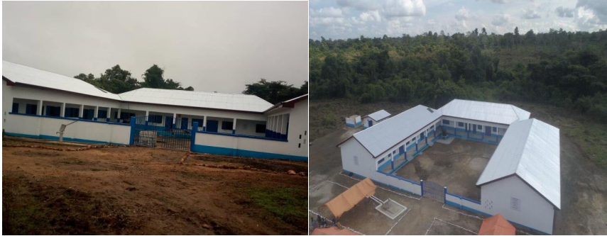
Figure 2 DONOR FUNDED CLASSROOM BLOCK AT NKRANKROM (ROTARY)
