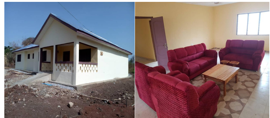
Figure 1 NURSES QUARTERS COMPLETED AND FULLY FURNISHED AT HANI (DDF FUNDED)
