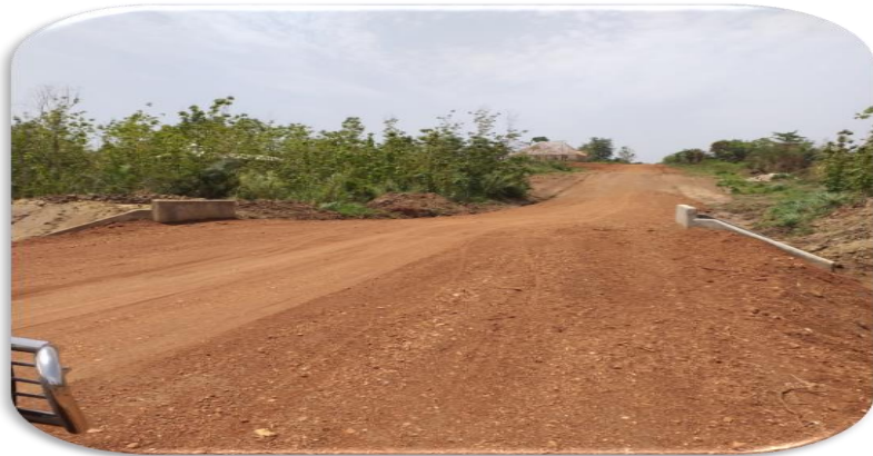
Construction of Odomase-Fiapre link road(6.5KM)
