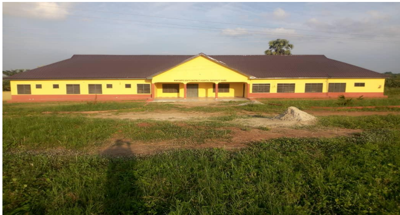
CONSTRUCTION OF 1NO. MATERNITY WARD AT JEMA DISTRICT HOSPITAL
