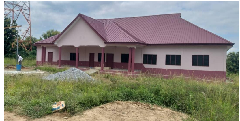
CONSTRUCTION OF FIRE SERVICE OFFICE COMPLEX AT JEMA
