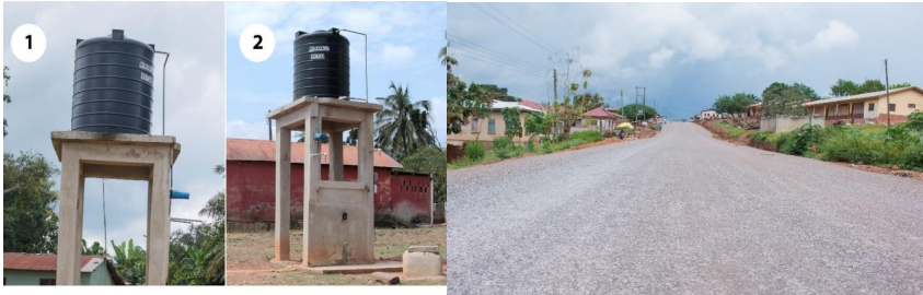
MECHANIZED 2 NO. BORE HOLE AT AHENBRONOM (1) AND ABURASO ZONGO (2) AT OYOKO - DACF
