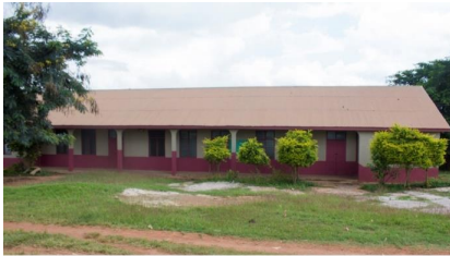
COMPLETION OF 1 NO. 3 UNIT CLASSROOM BLOCK WITH OFFICE AND STORE AT SEKYERE D/A JHS - DACF
