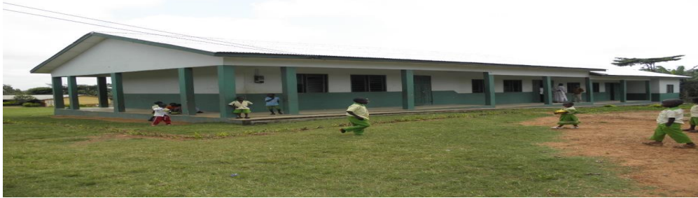
3-Unit classroom block @Nsuase Islamic Primary
