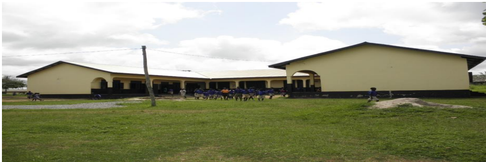
6-Unit classroom block @Benim
