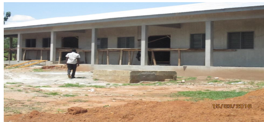
3Unit classroom block @ Nnobem (On-going)
