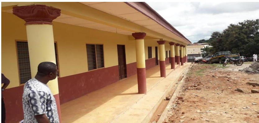
10. Construction of 1No. 3unit Classroom block at Meduma.
