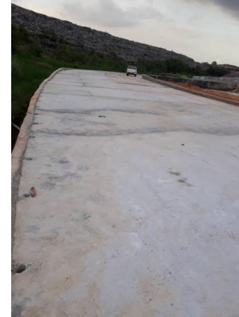
Figure 6: Newly constructed 945sq meter reinforced concrete ramps at Oti
