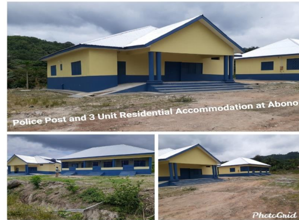
1 No. POLICE POST & 3 UNIT RESIDENTIAL ACCOMMODATION AT ABONO
