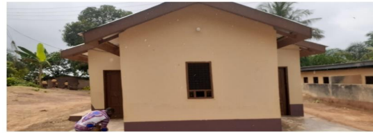
10 Seater Aqua Privy Toilet at Patrensa
