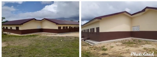
6 Unit Classroom Block at Apinkra
