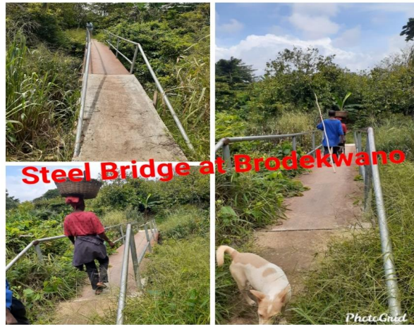
1 No. STEEL BRIDGE AT BRODEKWANO
