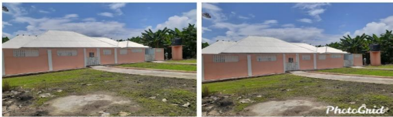
CHPS Compound at Pipie
