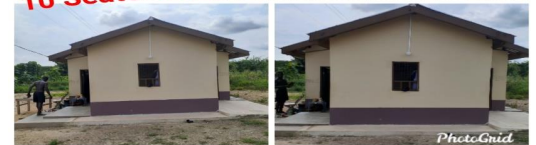
10 Seater Aqua privy toilet at Onwe
