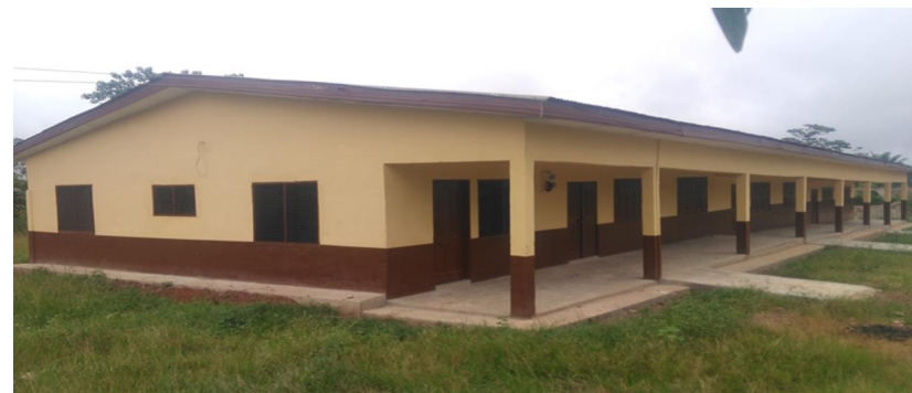
School Building at Binsere
