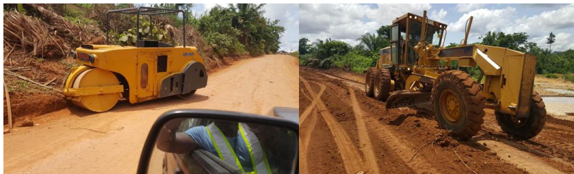
Reshaping of Road at Binsere
