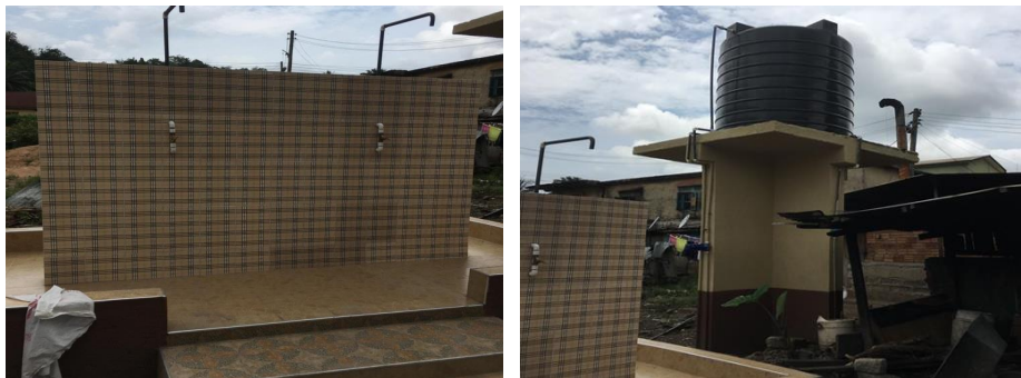
Mechanized Borehole at Wawasi
